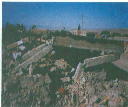
Photo 2-19: Collapse due to excessive sway deformation during 1997 Iran-Qayen Earthquake. Failure was due to pull-out of column longitudinal reinforcement from beam column connection.
