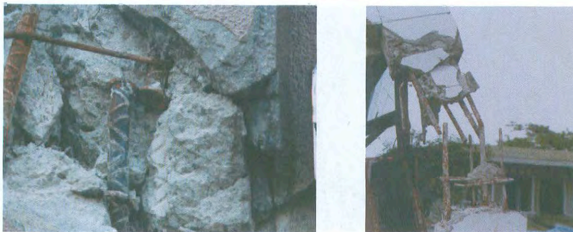
Photo 2-25: (Left) Gas pressure welding splice was fractured during the 1995 Hyogo-ken Nanbu Earthquake, Japan. (Right) Failure at lap splice in a building in Baguio during the 1990 Luzon Earthquake.
