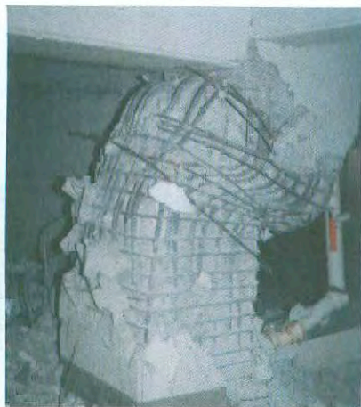
Photo 2-18: Flexural compression failure of columns in 1995 Kobe earthquake. Column had peripheral ties at 100mm centres in Motoyama Royal Condominium Building.
