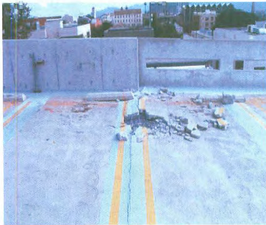
Photo 2-8: (Left) Buckled topping slab on precast diaphragm during the 1994 Northridge Earthquake. The mild tension reinforcement apparently yielded due to diaphragm flexure, then buckled as the unbonded prestressing reinforcement compressed the elongated mild reinforcement. (Right) Fractured diaphragm reinforcement at connection with structural wall. Source: W.G. Corley
