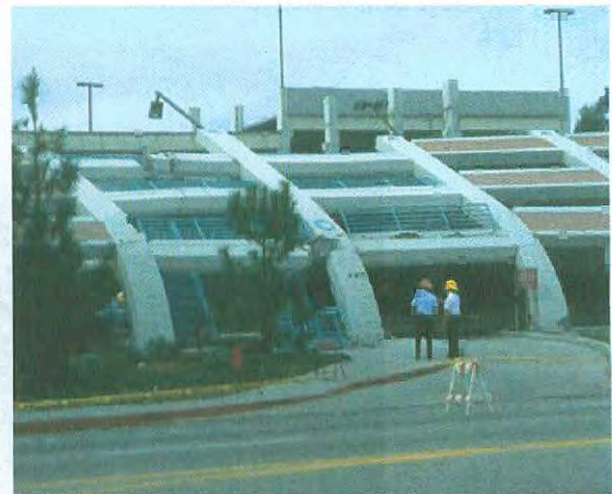
Photo 2-9: Consequence of column failures; (Left) Failure of interior "gravity" columns apparently led to (Right) progressive collapse of perimeter lateral force resisting system. 1994 Northridge earthquake. Source: NISEE
