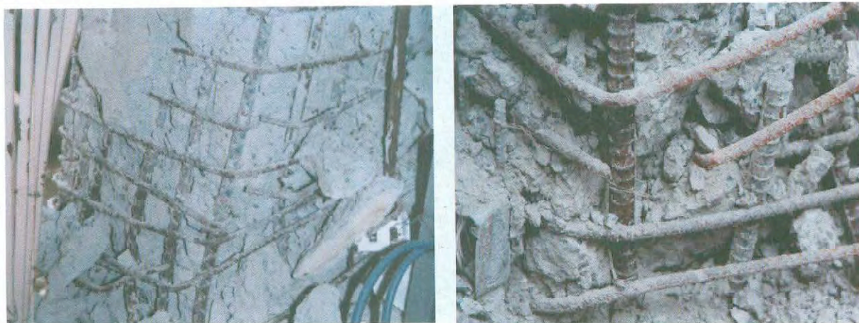
Photo 2-22: Shear failures in columns during the 1995 Hyogo-ken Nanbu earthquake. (Left) Opening of ties at a 90^\circ bend. (Right) Fracture of lateral reinforcement at the corner in a column.
