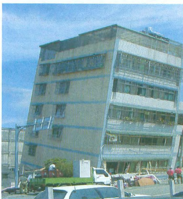
Photo 2-6: First-storey failure of corner building due to torsion in the 1999 Chi Chi Taiwan earthquake. Note open front and wall at the back. Source: NISEE
