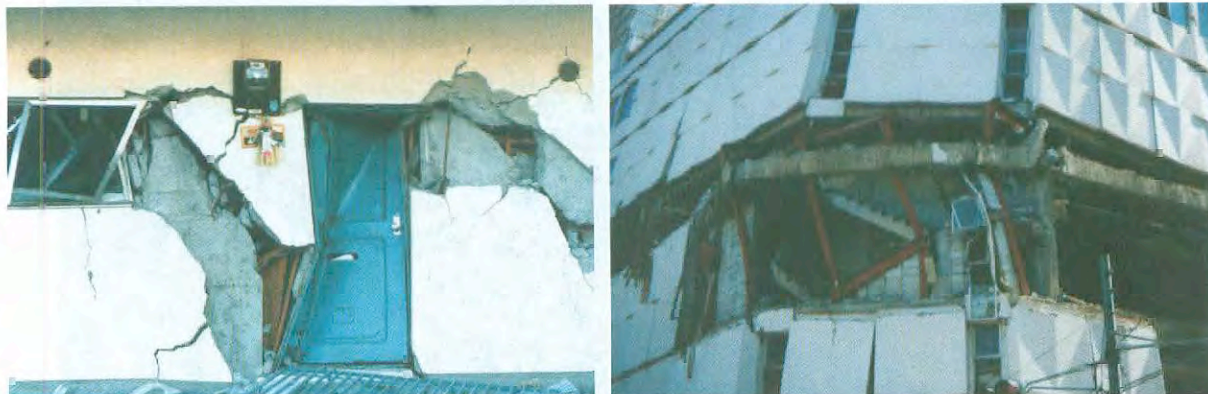
Photo 2-14: (Left) Damage of an entrance door and non-structural concrete partition walls due to large deformation in the 1995 Hyogo-ken Nanbu (Kobe) Earthquake, Japan. (Right) Fallen heavy precast concrete curtain walls in a building, Kobe City, in the 1995 Hyogo-ken Nanbu (Kobe) Earthquake
