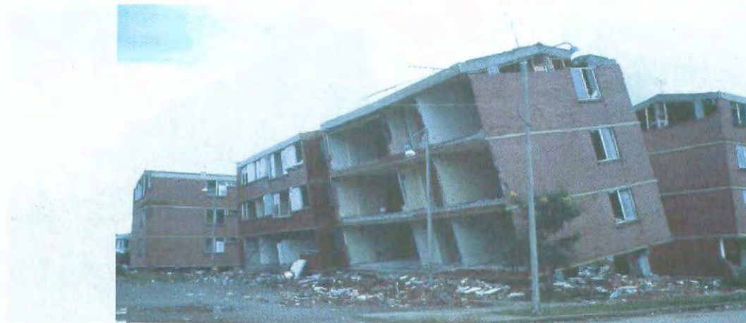
Photo 2-10: Twelve identical buildings collapsed when first storey stiff brittle masonry walls failed thus causing the reinforced concrete frame columns to fail in shear during the Popayan, Colombia, Earthquake of March 31, 1983.
