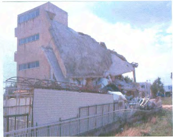
Photo 2-7: (Left) The damage occurred on the right side where the structural wall was discontinued in the first level on the right, while the structural walls were continued to the ground on the left (the 1978 Miyagi-ken Oki earthquake, Japan). (Right) Collapse of frames due to elevator shaft and staircase at one corner of the building plan by the 1999 Athens earthquake
