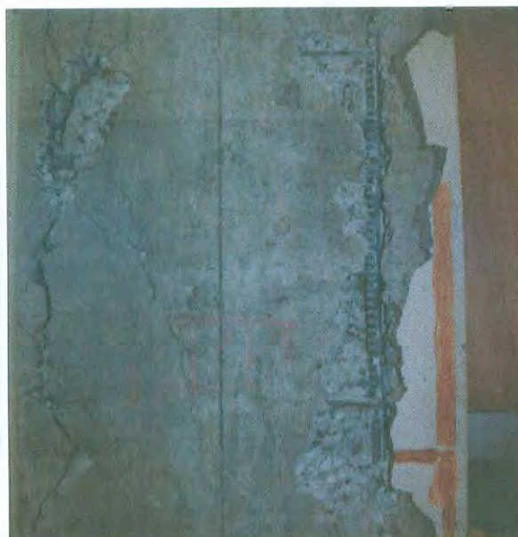
Photo 2-24: Bond splitting cracks were developed along the longitudinal reinforcement in columns of Namioka Hospital, Aomori, in the 1983 Mid-Japan Sea Earthquake; deformed bars were used with round-bar lateral reinforcement; concrete strength was low in this area due to poor coarse aggregates.
