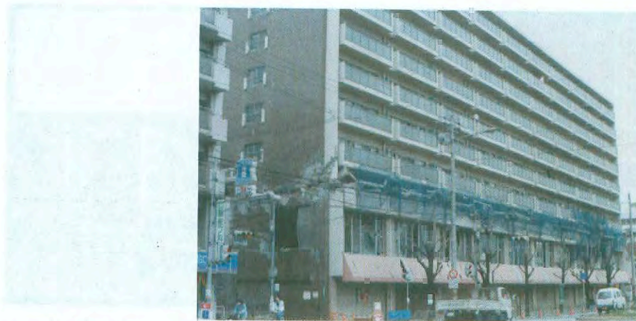
Photo 2-4: Condominium building collapsed in the third storey in the 1995 Hyogo-ken Nanbu (Kobe) Earthquake.
