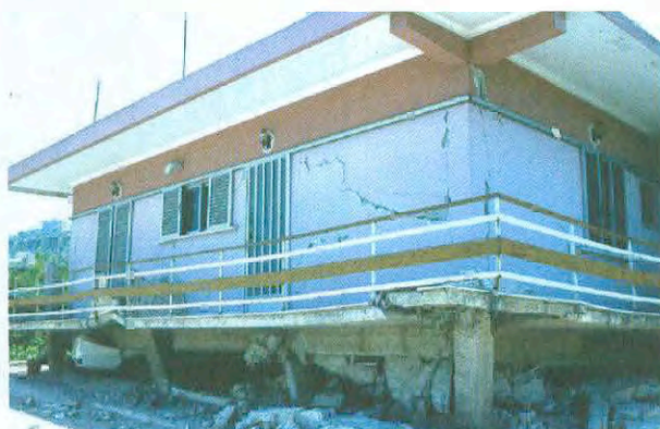
Photo 2-3: (Left) Rokko Building, Kobe, collapsed in the first storey in the 1995 Hyogo-ken Nanbu (Kobe) Earthquake, Japan. (Right) Two-storey building collapsed in the open ground storey in the 1995 earthquake in Aegion, Greece.
