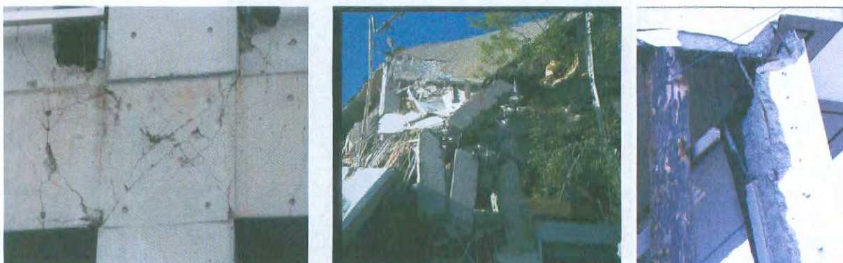
Photo 2-27: (Left) Beam-column joints of weak-beam strong-column building were heavily cracked in shear during the 1995 Hyogo-ken Nanbu, Japan earthquake. (Centre) Joint failures in older concrete frame in 1994 Northridge earthquake. Source: NISEE (Right) Diagonal failure of unreinforced corner column in 7-storey building in the 1986 Kalamata earthquake, Greece.
