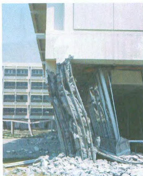
Photo 2- 2: Olive View Hospital, heavily damaged in the ground storey in 1971 San Fernando Earthquake, CA.
