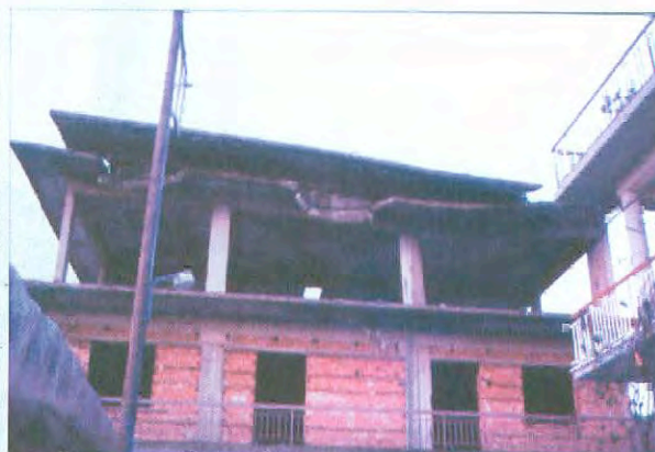
Photo 2-5: (Left) Collapse at third storey in 4-storey building in the 1999 Kocaeli earthquake in Turkey. (Right) Penthouse collapse in 5-storey building in the 1986 Kalamata earthquake in Greece.
