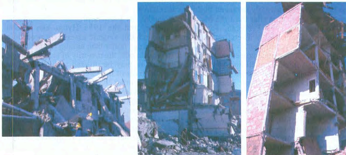
Photo 2-28: Examples of collapse of precast concrete buildings in 1988 Spitak earthquake in Armenia: (Left) Collapse of frame under construction in Leninakan. (Centre) Collapse of building in Spitak composed of wall panels with connections of plain cast-in-situ concrete and hollow-core slabs. (Right) Collapse of building in Leninakan, built of precast and in-situ infilled frame panels
