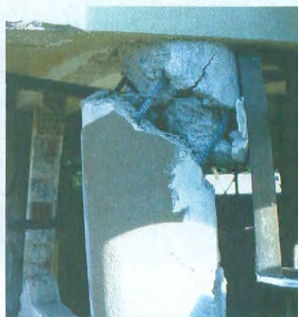
Photo 2-21: Column shear failures: (Left) in school building in Lazaro Cardenas, Mexico, during 1985 Mexico Earthquake. Spacing of the large-diameter ties was almost as wide as width of the column. Spalling of concrete was observed along longitudinal bars. (Right) in a building in 1986 Kalamata Earthquake, Greece; stirrups of plain bars were open and had no hooks or bents at the ends.
