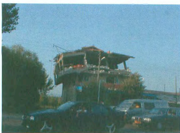
Photo 2-5: (Left) Collapse at third storey in 4-storey building in the 1999 Kocaeli earthquake in Turkey. (Right) Penthouse collapse in 5-storey building in the 1986 Kalamata earthquake in Greece.
