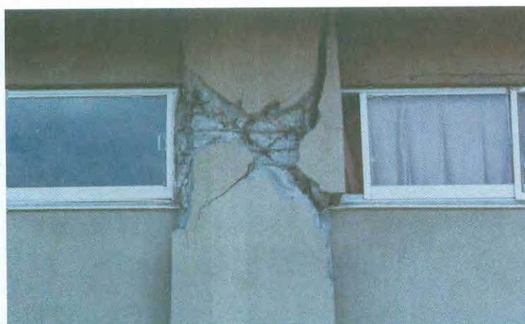
Photo 2-23: In Railway Technical High-school during the 1978 Miyagi-ken Oki Earthquake; non-structural but monolithically cast concrete walls restrained the deformation of a slender reinforced concrete column and caused the lateral deformation to concentrate in a short length
